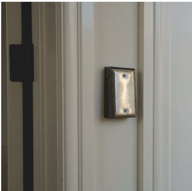
The electronic door opener is placed within easy reach of the son's wheelchair.
