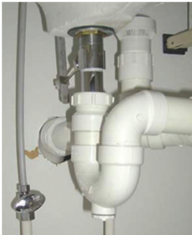
Air admittance valves (AAVs) eliminate the need for many piping and roof penetrations.
