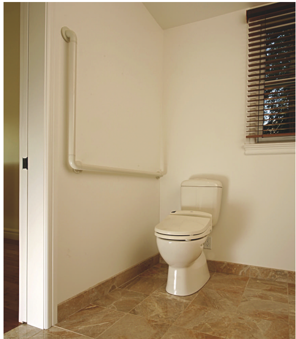
The master bath has a chair-height toilet, room for the wheelchair to maneuver and an extended grab bar.
