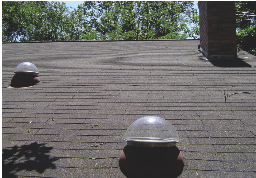
Tubular skylights let light shine into windowless spaces like interior bathrooms or hallways.
